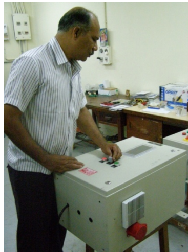
Control panel fabrication
